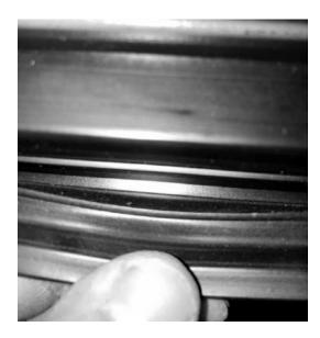
10. After installation of the overlay panel is completed, verify that the gasket is completely sealing around the cabinet frame. If installing panels onto drawer models (-6), repeat installation process for second drawer face. Installation is now complete.
