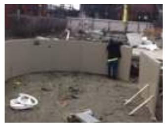
smooth liner installation and a flush top seat fit. Use a level to make sure that the pool walls are both plumb and level.
