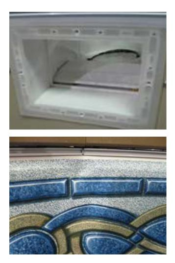
The weight of the vinyl pulling down will keep the bead in the coping. Make sure that the points around the perimeter of the liner floor match up with the panel joints of the pool wall. All wrinkles must be removed before filling with water.
