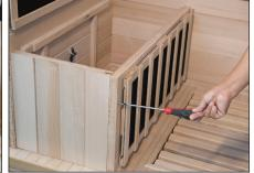
7. Plug in all bench heater plugs into wires from back wall. Make sure connections are tight. Attach the BENCH SEATS with (2 ea.) 2" SCREWS in pre-drilled holes into BENCH SUPPORT.
