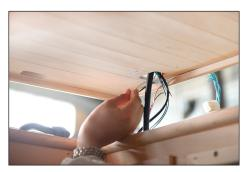
\*While placing the roof over the sauna, feed each of the heater cables on side & back walls, and the wire harnesses and power plug in back left corner, through corresponding holes on perimeter of roof.
