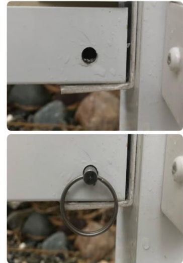
Figure 8 Hole for Clevis Pin and Clevis pin installed
