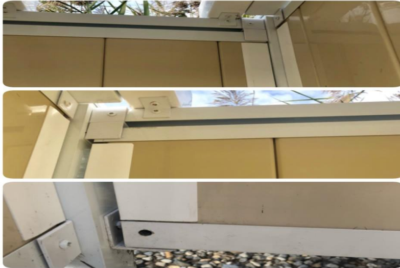
Figure 9 Double Header (U channel)
