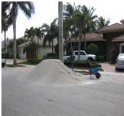
\frac{3}{4} " to \frac{1}{4} " Primary Base Drain Rock
